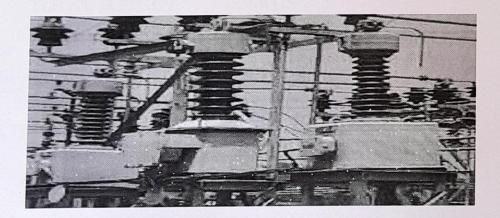
The secondary voltage of the PT is generally 110 V. In an ideal potential transformer or voltage transformer, when rated burden gets connected across the secondary; the ratio of primary and secondary voltages of transformer is equal to the turns ratio and furthermore, the two terminal voltages are in precise phase opposite to each other. But in actual transformer, there must be an error in the voltage ratio as well as in the phase angle between primary and secondary
