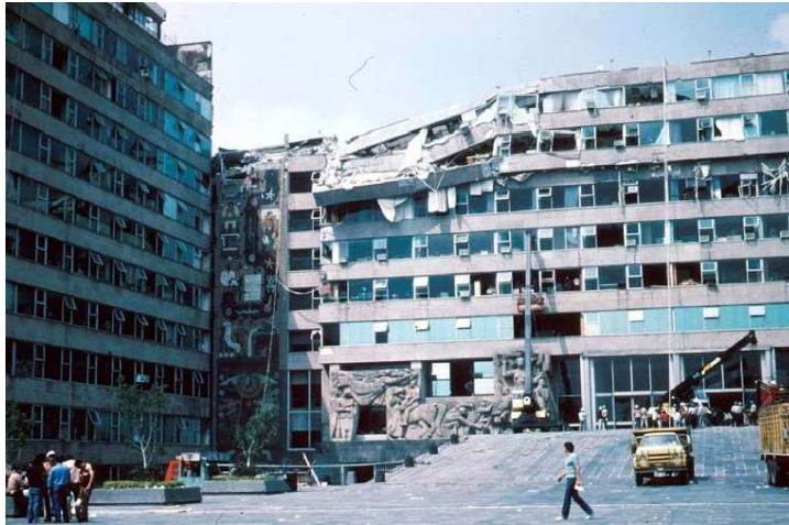
Figure 1.3 Damage to Reentrant corner and Upper stories of the Ministry of Telecommunications Building in Mexico City after the 1985 earthquake.
