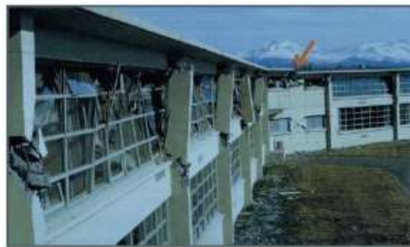
Fig-2: Damages caused to the Roof Diaphragm at the Re-entrant Corner of West Anchorage High School, Alaska, during the 1964 earthquake
