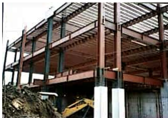
FIG. 1.4 COMPOSITE COLUMN WITH CONCRETE BEAM
