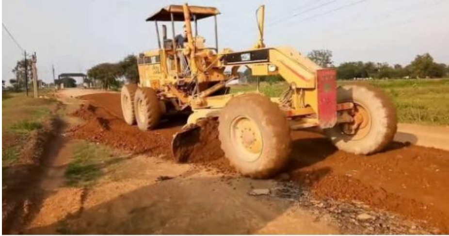
Fig 1.2.1.3: Laying sub- base course
