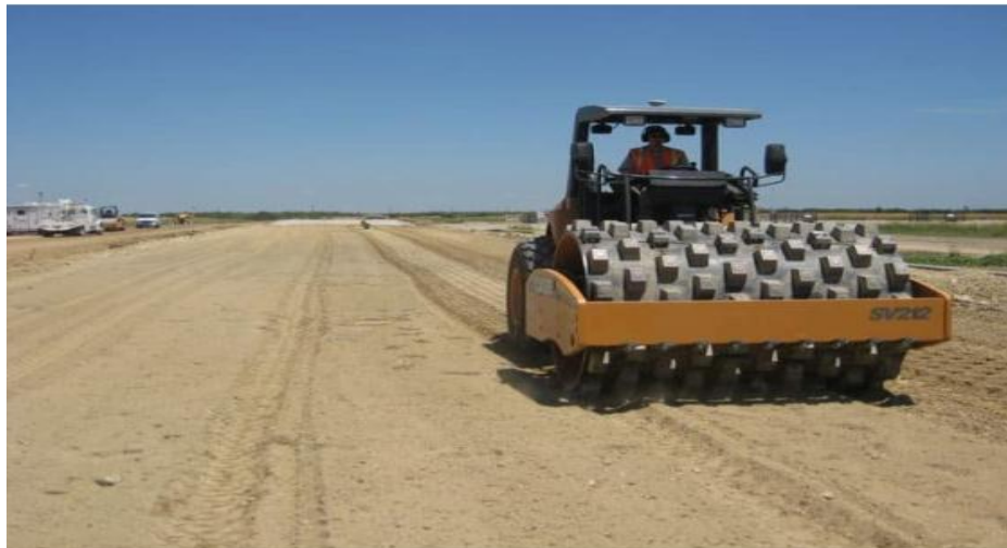
Fig 1.2.1.2: Compacting sub-grade
