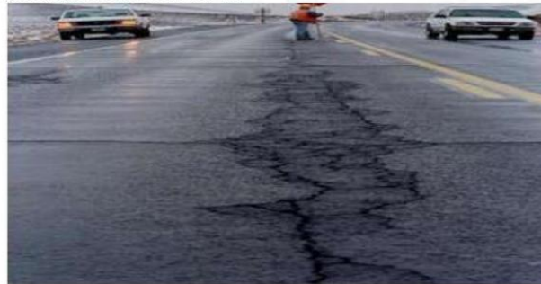
Fig 1: Cracking caused by stripping at the bottom of HMA layer
