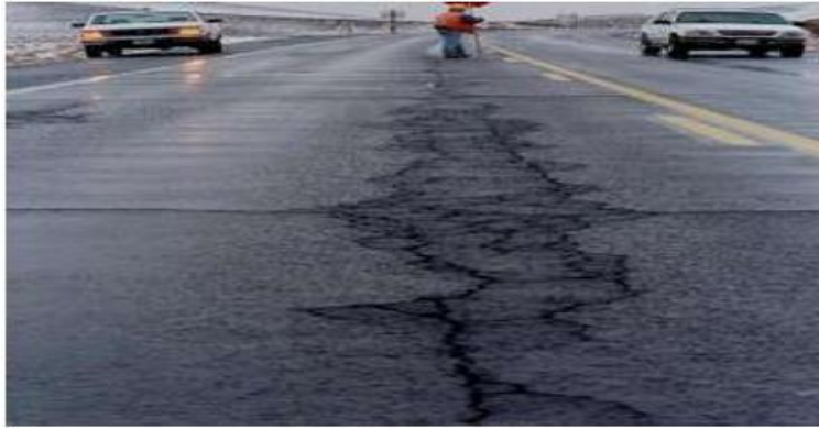
Fig 1.4(a): Cracking caused by stripping at the bottom of HMA layer
