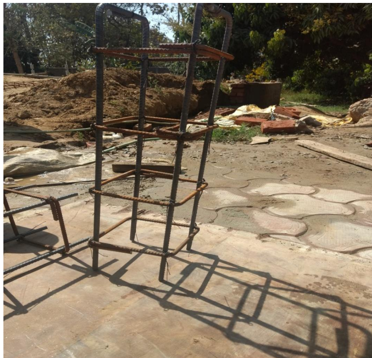
Fig 3.11 Phase I Reinforcement of Column
