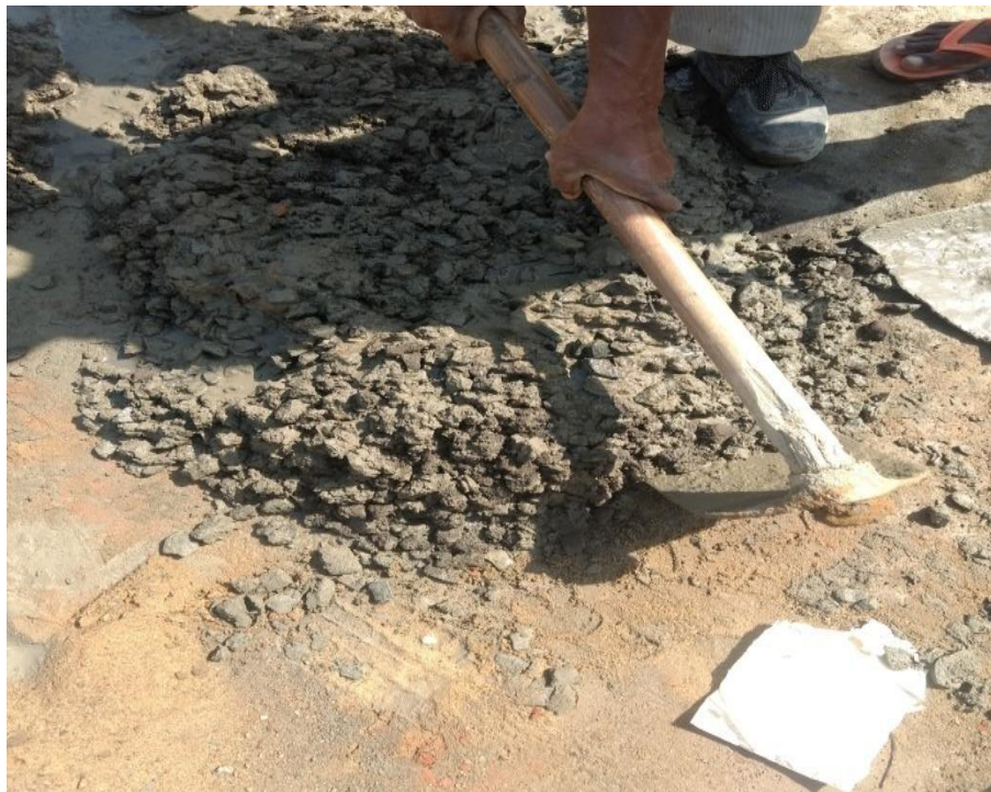
Fig 3.13 Mixing of Concrete
