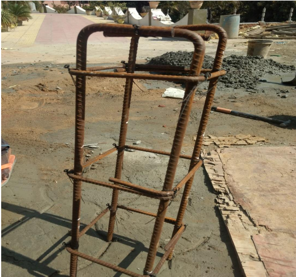
Fig 3.12 Phase II Reinforcement of Column
