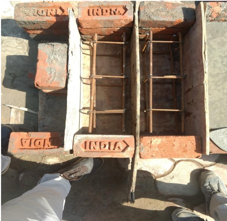
Fig 3.14 Casting of short column with timber frame
