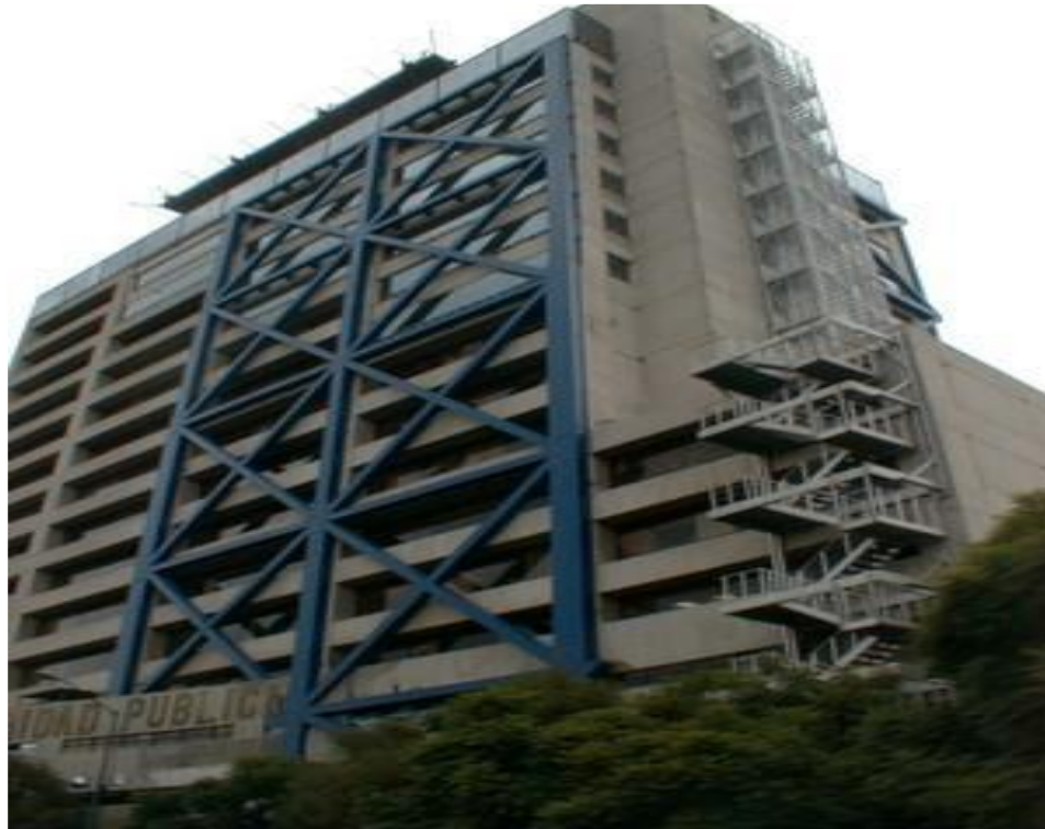
Figure 1.3- RC Residential Building with bracing
