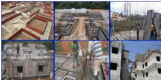
Fig.3 – A Typical working of a Monolithic Concrete Construction Technology
