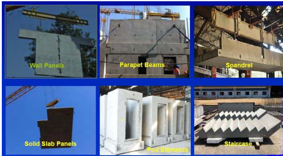
Fig.2 – Parts of prefabricated structure
