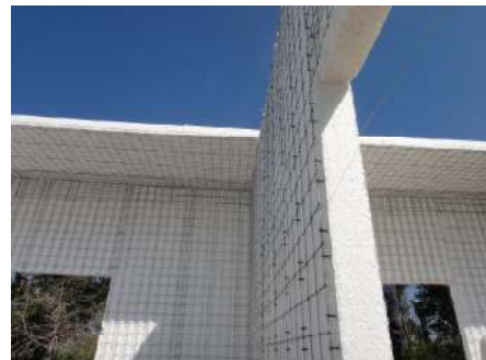
Fig.6 – A Typical working of a SIP panels
