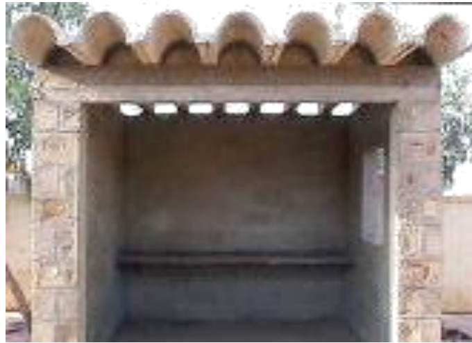
FIG.2 FERROCEMENT BARREL SHELL ROOFING SYSTEM
