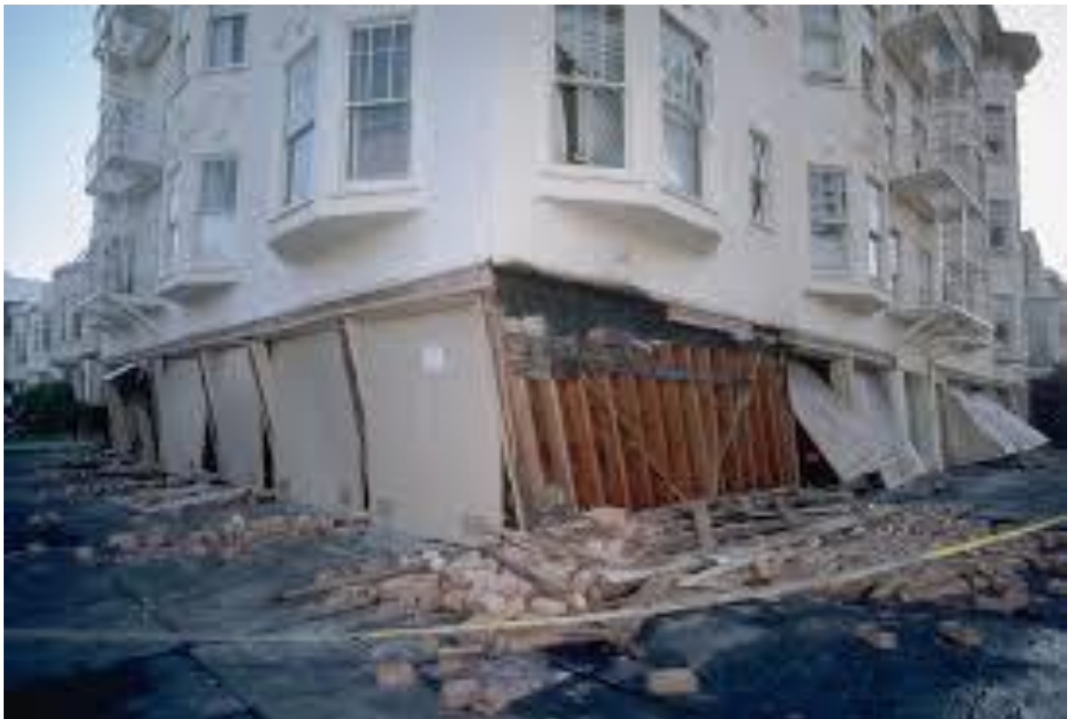
Figure 1.1 Failure of OGS Building Due to Buckling
