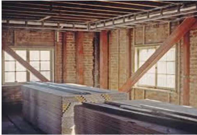
Figure1. 2 bracing in masonry building
