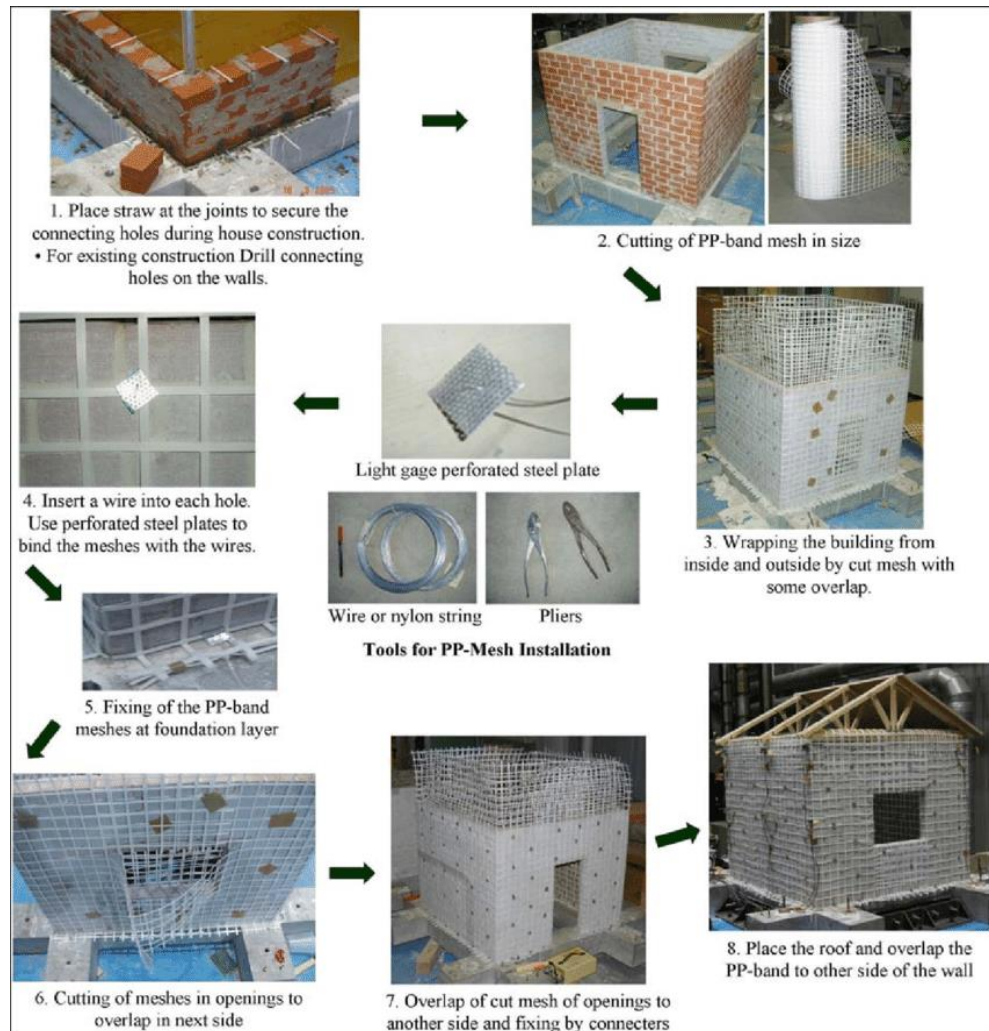
Figure 1.11 – PP mesh installation
