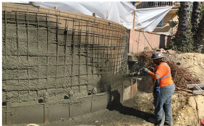
Figure 1.6- Shotcrete on the site by nozzal
