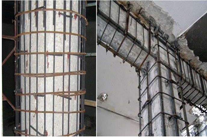
Figure 1.15- Concrete jacketing
