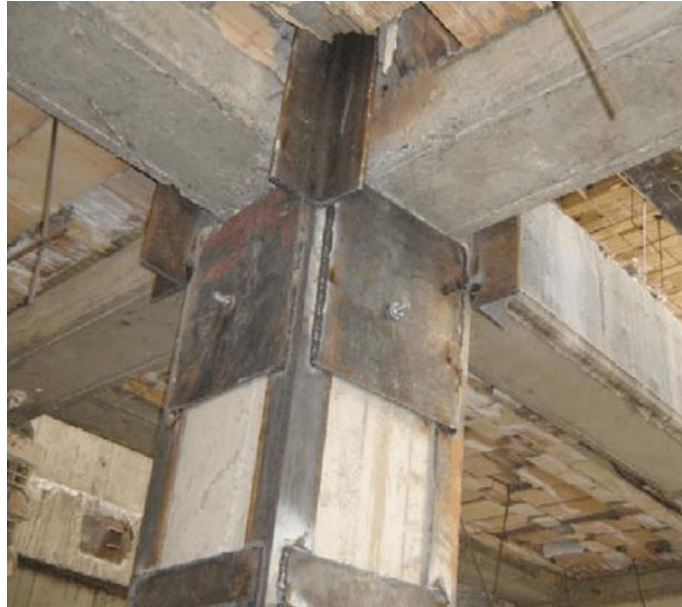
Figure 1.14- steel jacking
