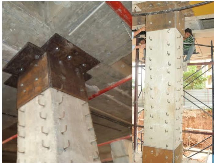
Figure 1.16- Steel jacketing
