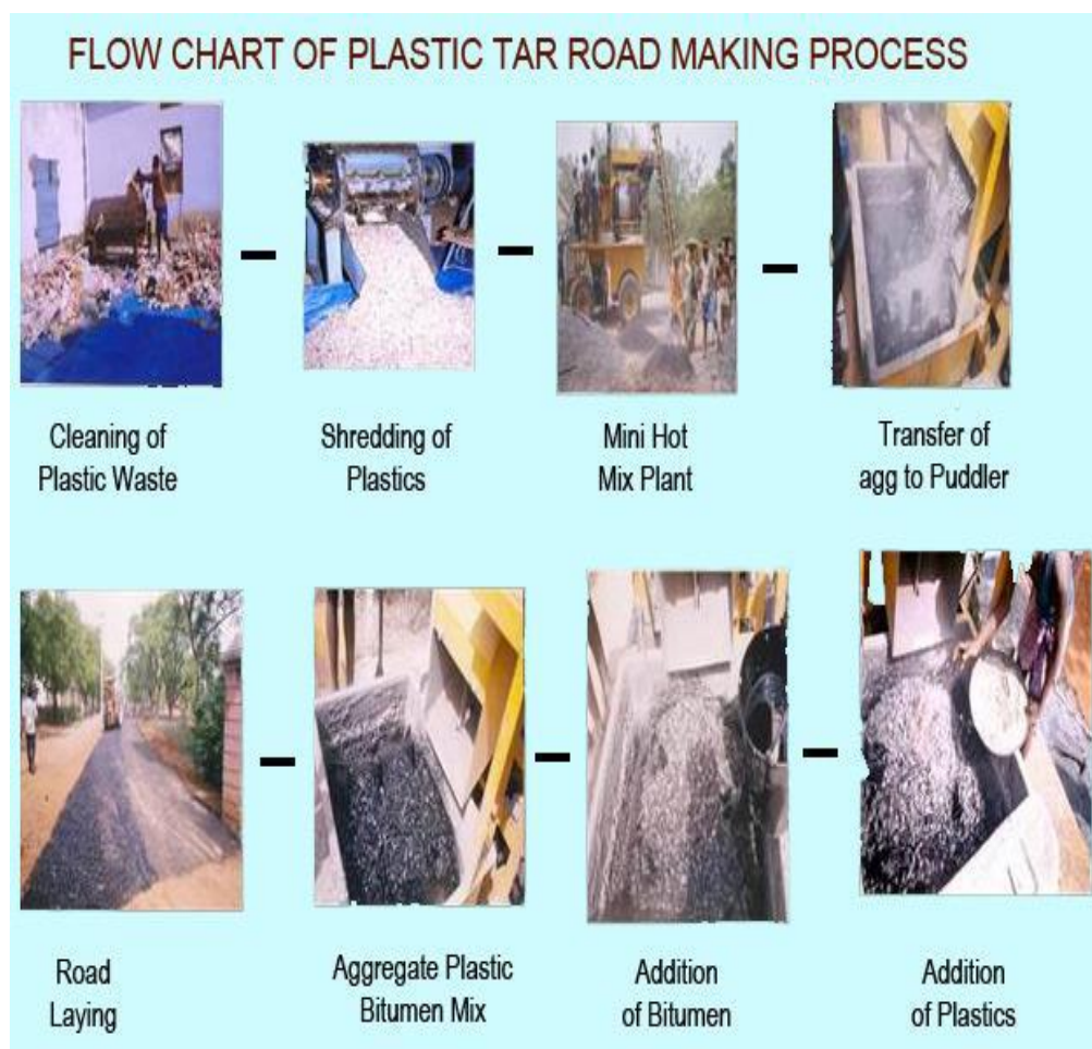
Fig. 3.7 Preparation of Plastic Coated Aggregate
