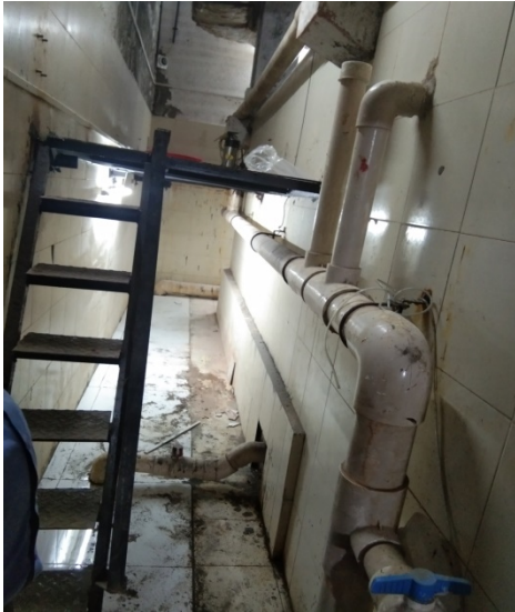
PIPE DIA11CM FROM FILTRATION TO OVERHEAD TANK
