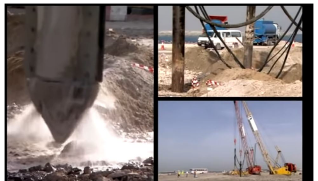
VIBRO COMPACTION METHOD
