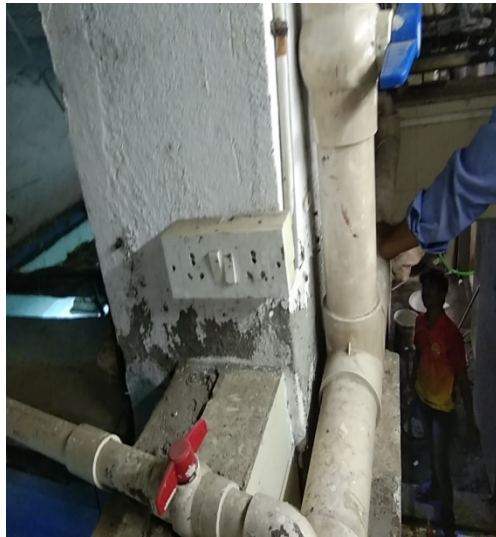
PIPE DIA 9CM FROM OVERHEAD TANK TO DISPLAY TANKS
