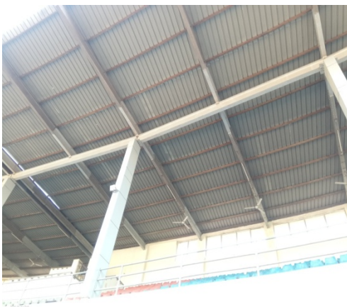
MILD STEEL FRAMED STRUCURE SHED
