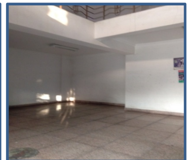
COMMON AREA FLOORING 15MM THICK GRANITE STONE IS USED FOR FLOORING
