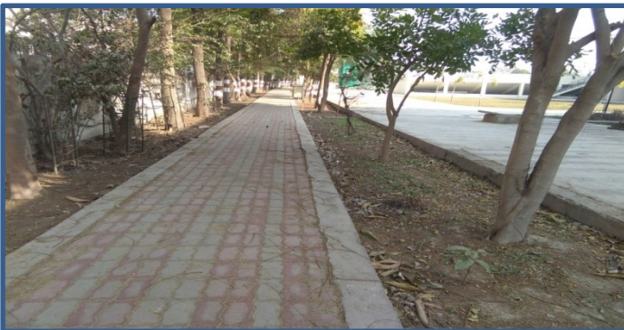
CONNECTING PATHWAY PAVED BY CEMENT BRICK
