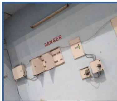
•MCB FOR LIGHTING •SKY BLUE PAINT IS USED FOR WALL FINISH
