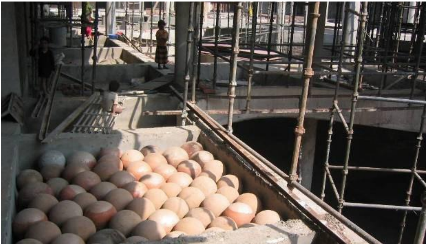
Image showing the use of matkas in the roof slab of Pearl Academy of Fashion during the actual construction.
