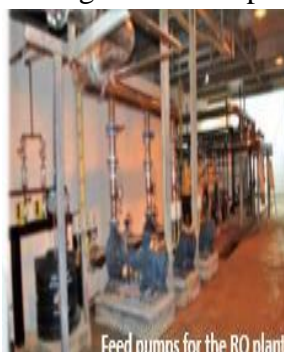
Feed pumps for the RO plant
