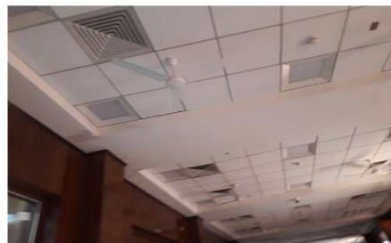
CEILING OF JUDGE CORRIDOR
