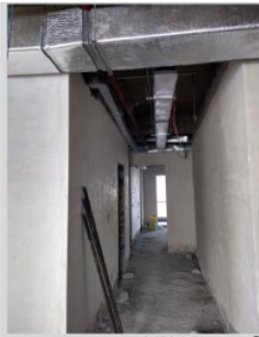
VRV Ducts & Sprinklers
