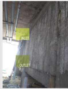
Water Tank (at service floor)
