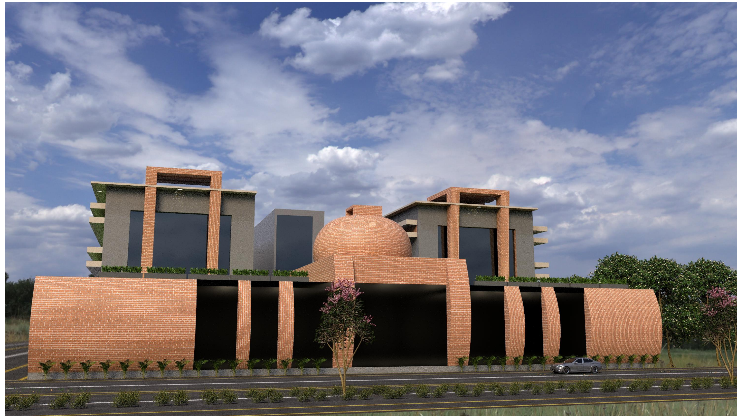
HOSPITAL BLOCK FRONT VIEW
