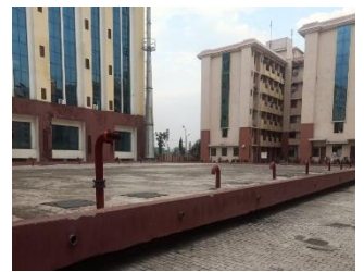
UNDER GROUND WATER TANK
