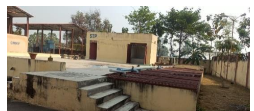
SEWAGE TREATMENT PLANT
