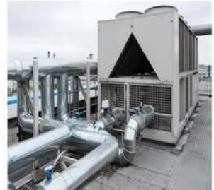
FIG: ROOF TOP CHILLAR PLANT
