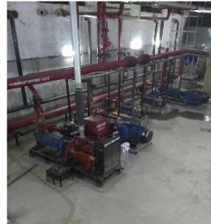
Pump Room (With Jockey Pump, Main Pump, DG etc.)
