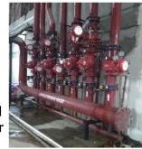
Sprinkler Line (for various Floors with PRVs)
