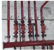
Hydrant Line (for various Floors with PRVs) (Pressure- 3-4 kg)
