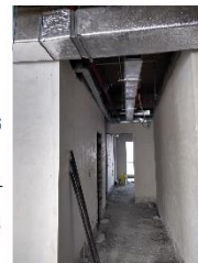
VRV Ducts & Sprinklers
