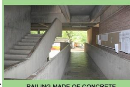
RAILING MADE OF CONCRETE
