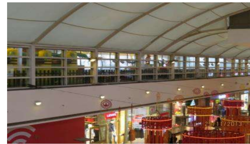
Linear Shaped Skylight- Running all along the mall. Covered with same material as atrium. Linear Skylights.
