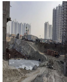
RAFT FOUNDATION CONSTRUCTION FOR TOWER-4
