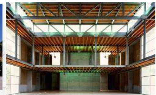
LIBRARY WITH COLUMN FREE AND STEEL BEAMS
