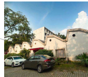
Zigzag roof are provided in the workshop for natural light ventilation.
