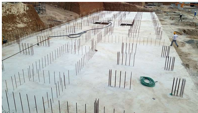
P1. FOUNDATION RAFT WITH WALLS PICTURE STARTER BARS FOR PRECAST COLUMNS
