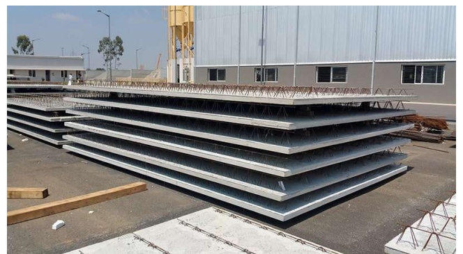
PICTURE 13. STACKING OF HALF SLABS
