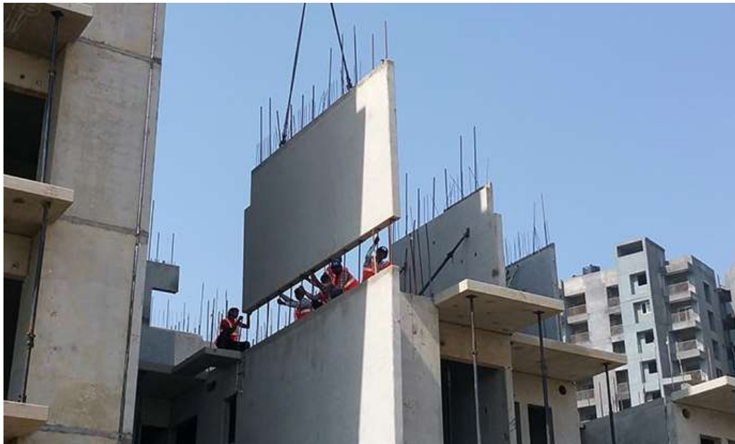
PICTURE 6. ERECTION OF LOAD BEARING PRECAST WALL PANEL
