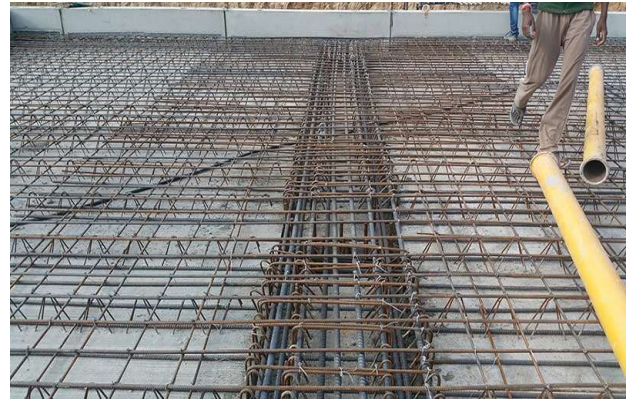
P4. EXTENDED BASEMENT STRUCTURE WITH PRECAST HALF BEAMS AND HALF SLABS
