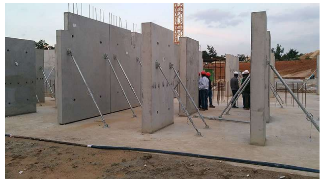
P2. BASEMENT PRECAST WALLS AND COLUMNS
