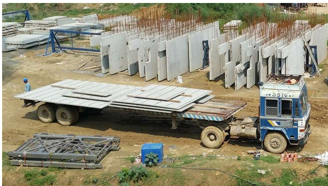
PICTURE 16. TRANSPORT OF PRECAST SLABS
