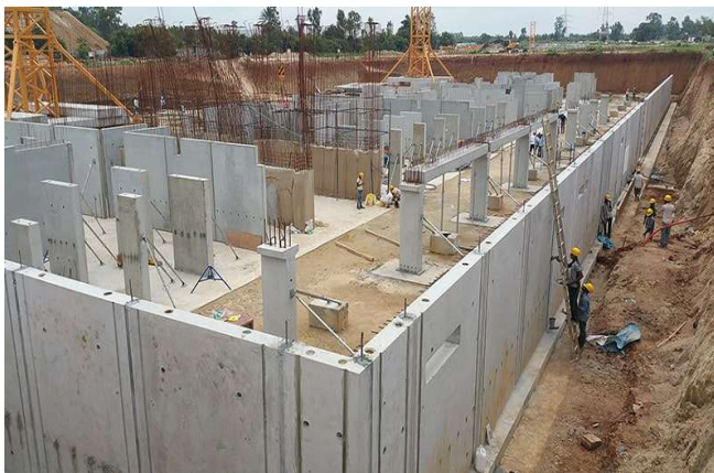
P 5. BASEMENT STRUCTURE WITH PRECAST RETAINING WALLS
