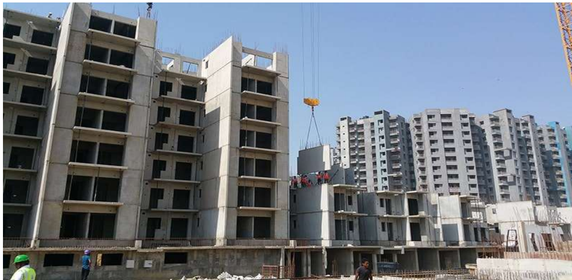
P3-A. PRECAST CONCRETE LOAD BEARING STRUCTURE ON TOP OF BASEMENT
