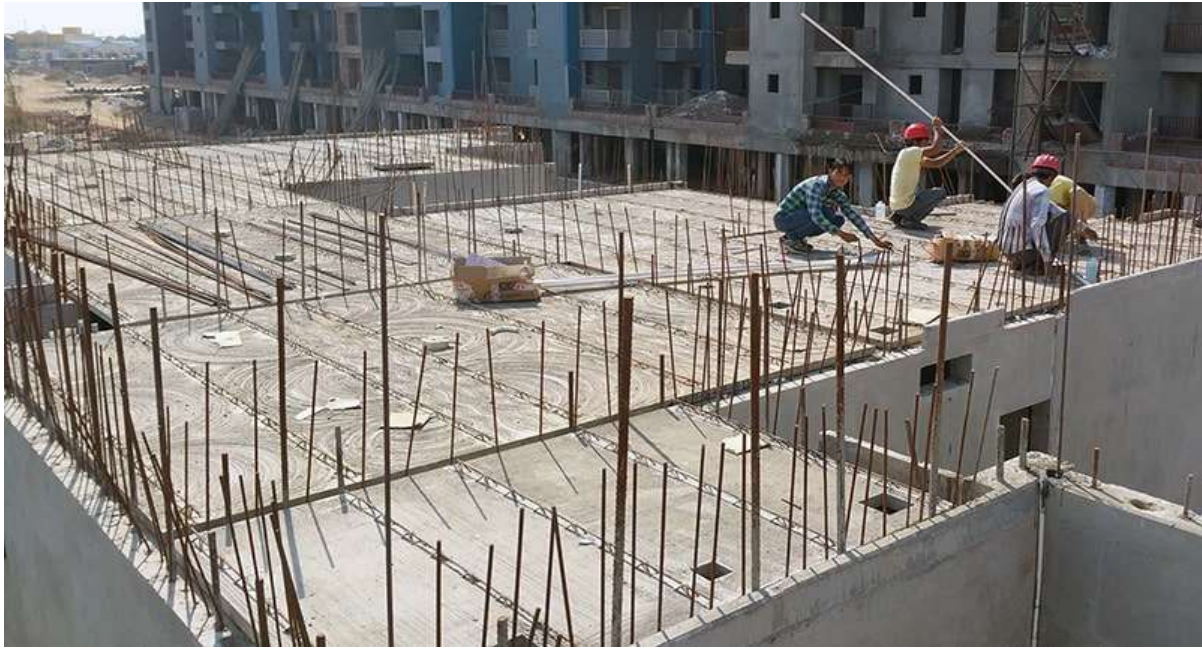
PICTURE 4. PRECAST HALF SLABS WITH LATTICE GIRDERS
