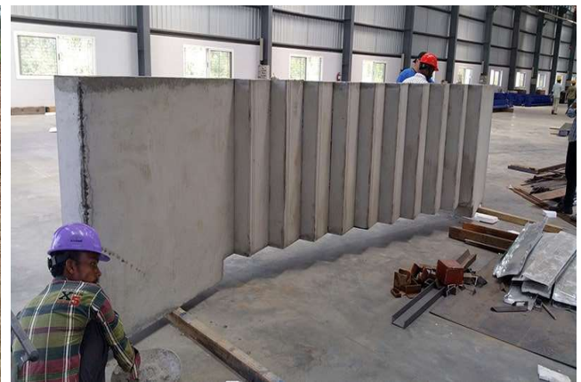
PICTURE 6. PRECAST STAIRS WITH ATTACHED BOTTOM AND TOP LANDINGS
