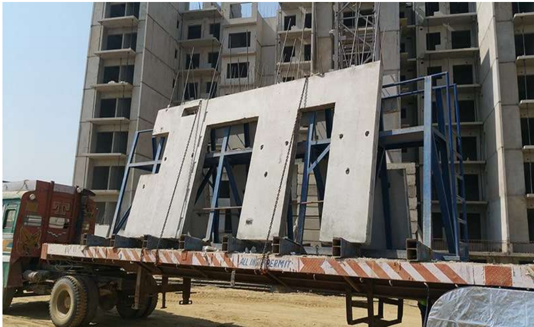
PICTURE 15. TRANSPORT OF PRECAST WALL PANELS
