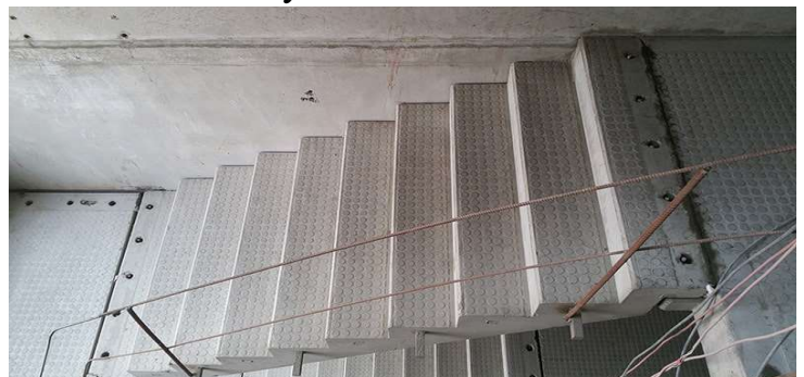
PICTURE 8. PRECAST STAIRCASE WITH LANDINGS AND STAIR FLIGHT
