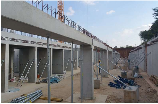
P3. EXTENDED BASEMENT STRUCTURE WITH PRECAST COLUMNS AND HALF BEAMS
