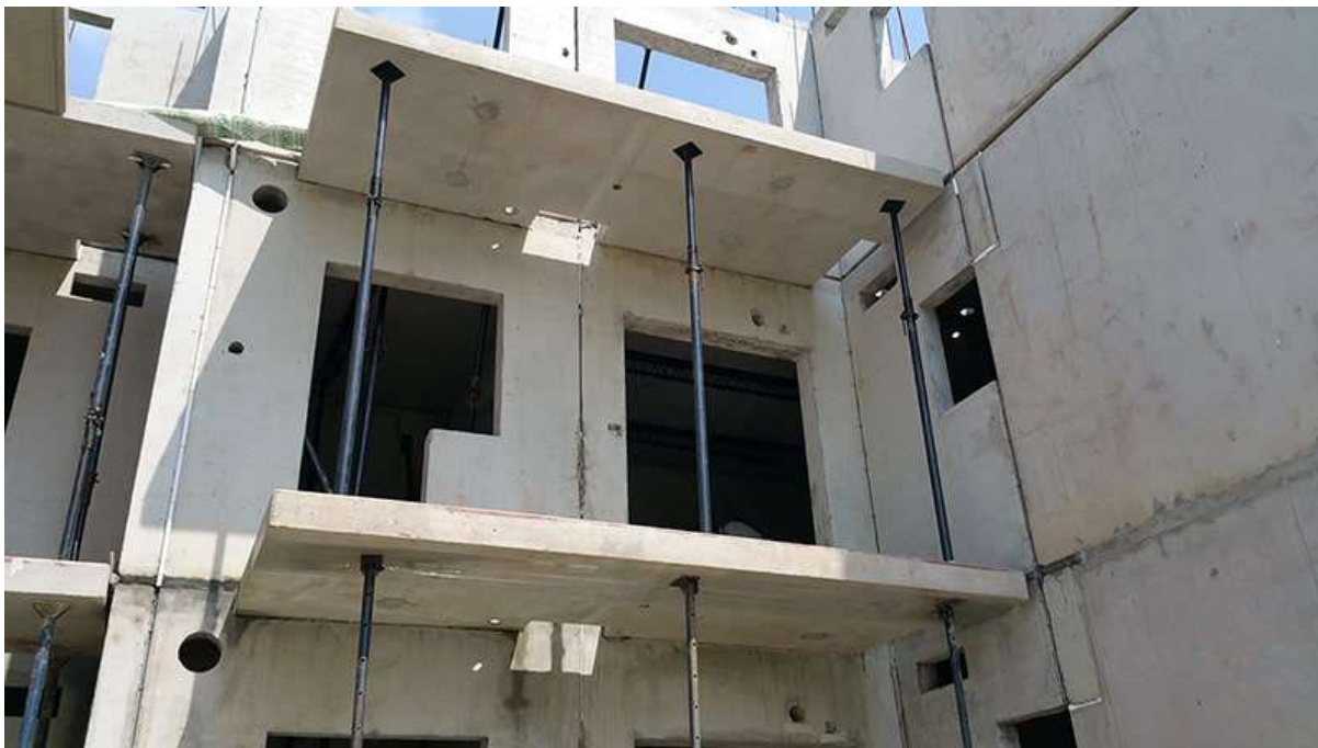
PICTURE 5. CANTILEVER PRECAST BALCONIES
