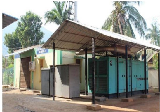
Generator room for flood lights.
