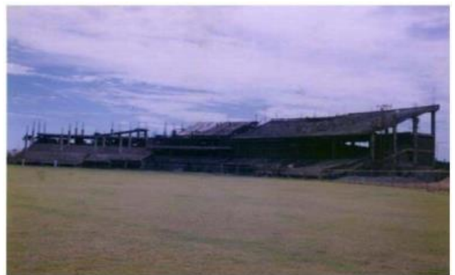
SECOND TIER CONSTRUCTION STAGE
