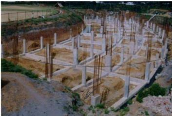
PLINTH BEAM CASTING
