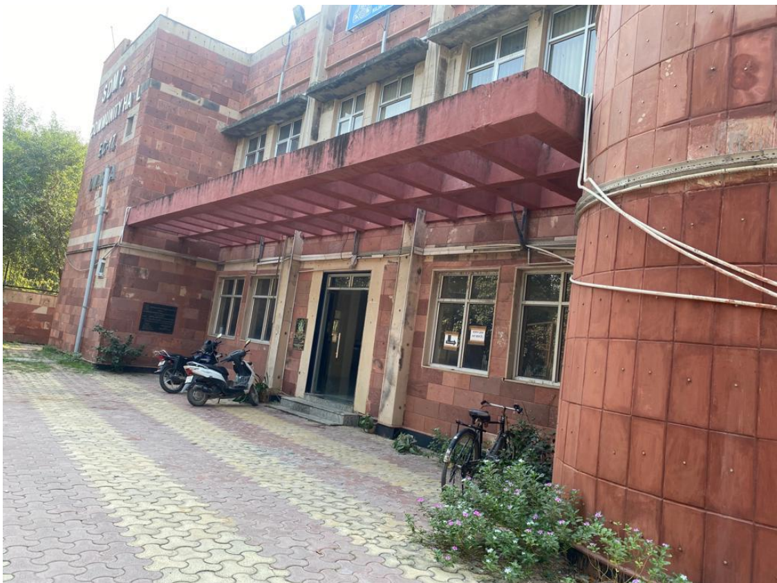
(Fig.119 ) porch which is not even protect rain, sunlight and have an heavy rcc structure.
