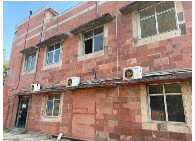
(Fig.112 &113) Elevations of sdmc office with plane stone stone cladding and normal openings.
