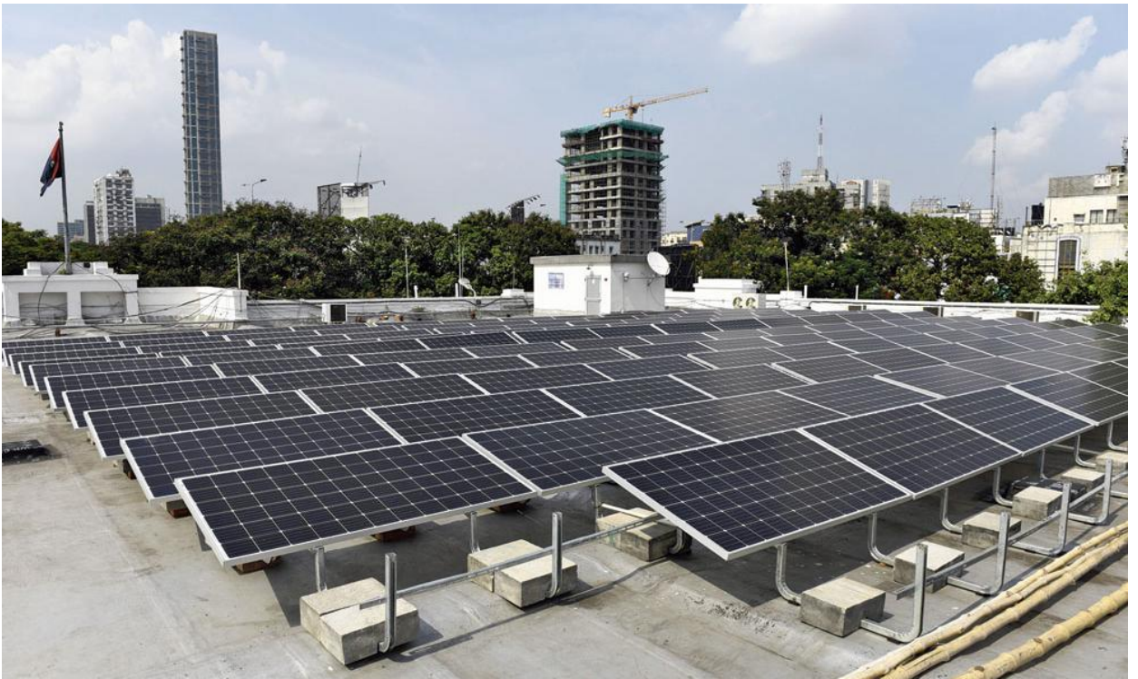
(Fig.120) Solar panels on terrace which reduces the electricity bill and aslo a power backup for the building A Sustainable Architectural point.
