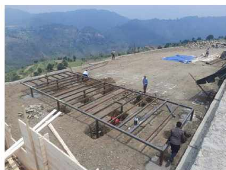
ongoing site-work isolated footing
