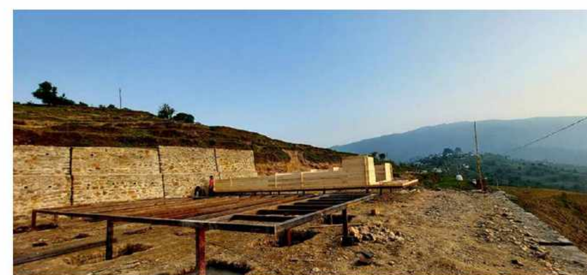
cut and fill has done on the site. MS square pipe frame has been developed at site for making plinth of wooden structure resting on it.
