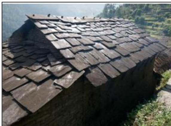
Figure 23: Stone Roofing
