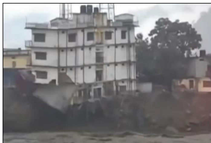
Figure 2:RCC structure just before the collapse
