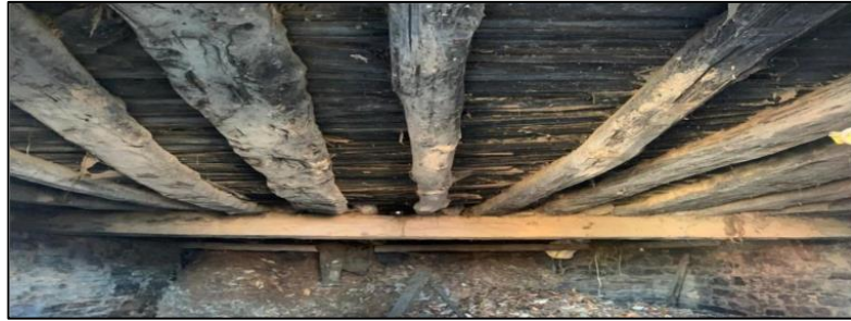
Figure 24:Roof supported on wooden beam and batten
