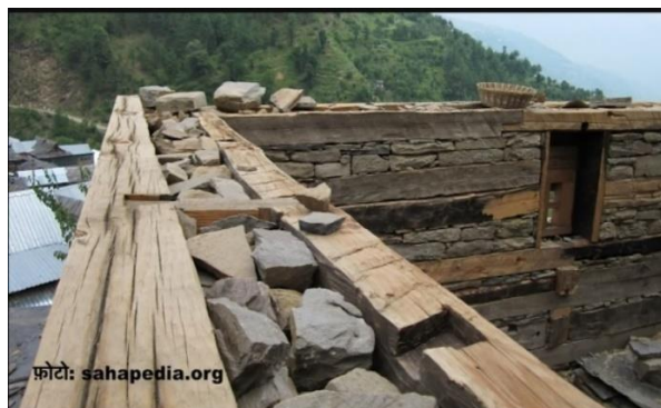
Figure 18: two parallel cross-beams held a dovetailed timber
