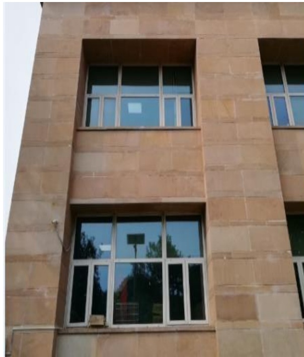
Figure 3.10:Fenestrations with double glazing (Source:Author)
