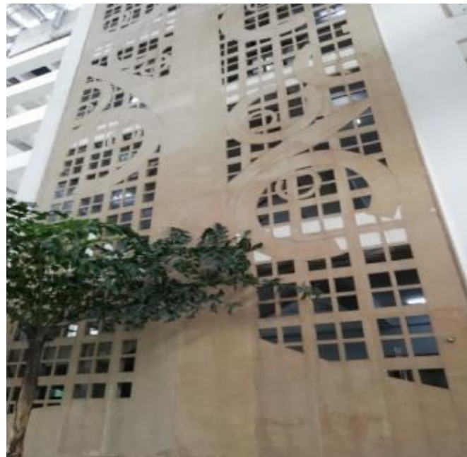
Figure 3.15:Stone jalis providing cross ventilation through staircase (Source:Author)
