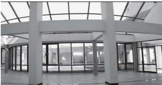
Fig. 20 North light roof used to naturally light the entire green technology center
