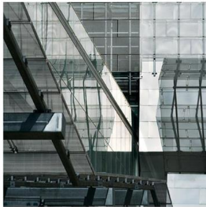
Fig. 14 Staggered windows with steel structure
