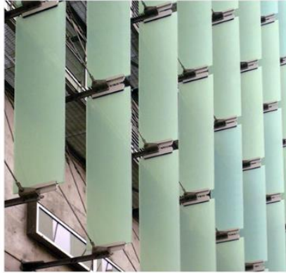
Fig. 11 Steel cables and metal clips with fins
