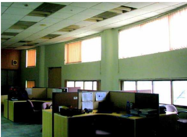
Fig. 20 North light roof used to naturally light the entire green technology center
