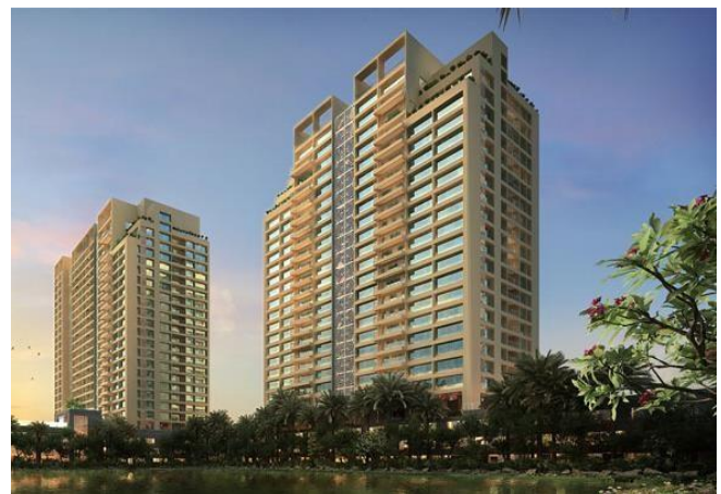
UTALIKA:- Location:Kolkata, West Bengal Under Construction
