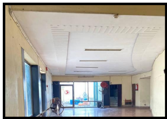
PLYWOOD CEILING AT SIDEWAY OF AUDITORIUM
