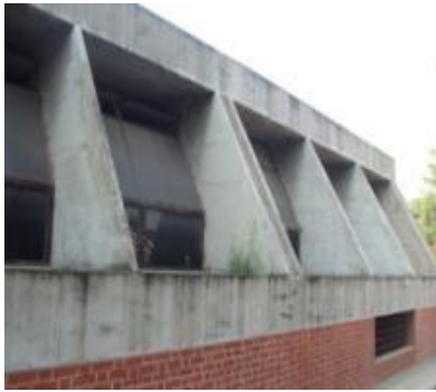
DESIGN OF THE OPENINGS TO GAIN THE MAX. SUN SHINE AND VENTILATION
