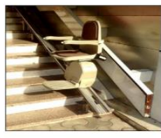
Figure 7-18: Platform chair lift and platform lift
