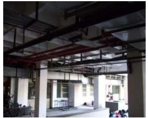
Fire hydrant pipes under false ceiling.
