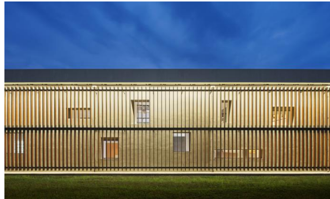
south elevation: double skin with compressed bamboo louvers and random voids
