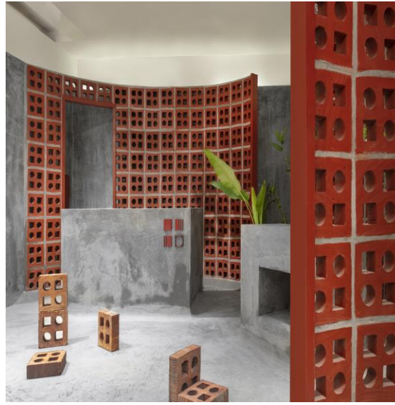
a series of curving walls made of terracotta bricks give way to a viewing gallery
