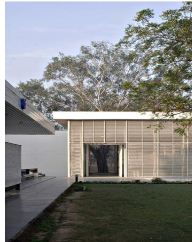
Front View, Jamia Art Gallery The Front view pictures a tree as the entrance opens to show through the space.
