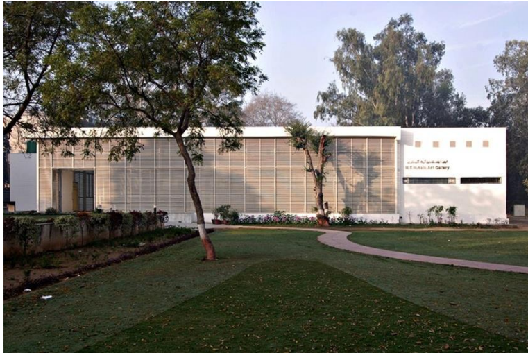
Front view of the Gallery M.F Hussain's Art Gallery, situated amid sprawling greens, looks its best in the daylight. Exterior, louvers, Elevation
