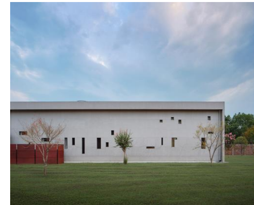
north elevation: the concrete is decorated with a pattern of cedar planks
