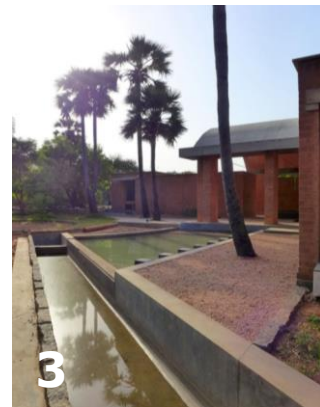
In response to the hot and humid climate, the open array of piers funnel coastal breezes into the building ensuring thermal comfort without air-conditioning or fans.
