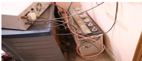
Figure 3.1(d) Connection between Solar Inverter and Solar Battery Source : Author
