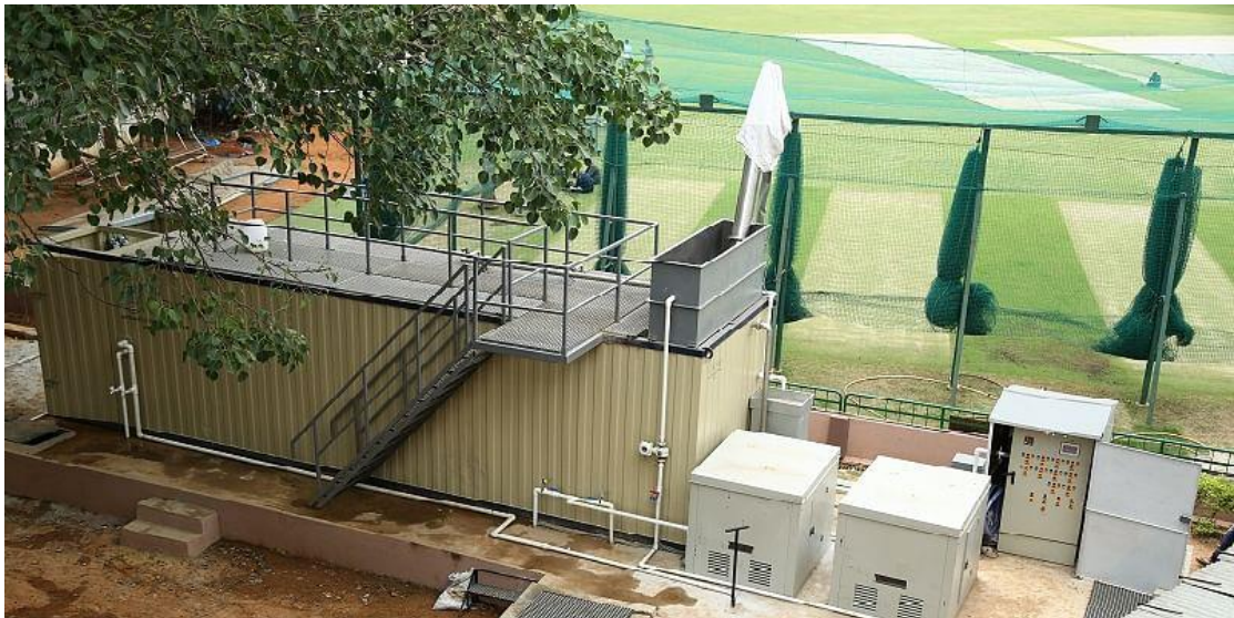
Figure 2.2 (d) STP installed at Chinnaswamy stadium Source : Author
