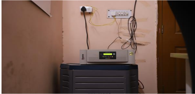
Figure 3.1(e) Connection between Solar Inverter and Solar Battery Source : Author
