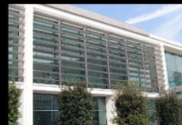
LOUVRES IN COMBINATION WITH GLASS ON THE SHOPS AS SHADING DEVICES
