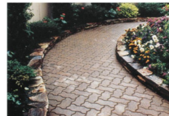
INTERLOCKING TILES AT THE PATHWAY CONNECTING WORKSHOPS AND DORMITRY
