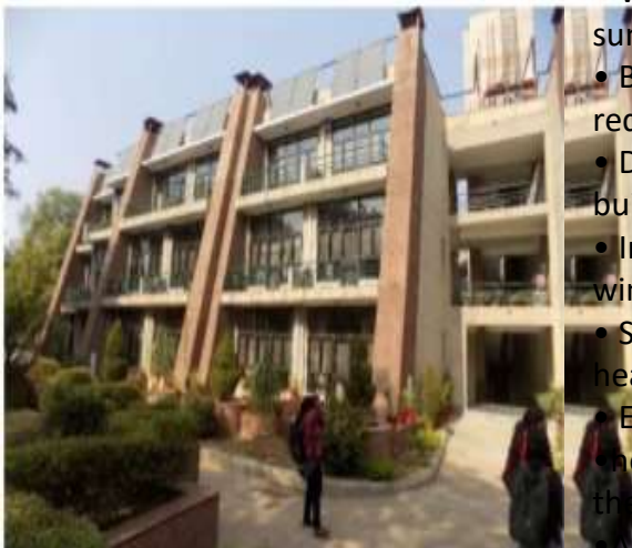
South view of facade
