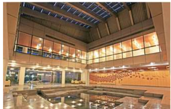
solar photovoltaic panels form the roof of the atrium of the learning centre , generating green power
